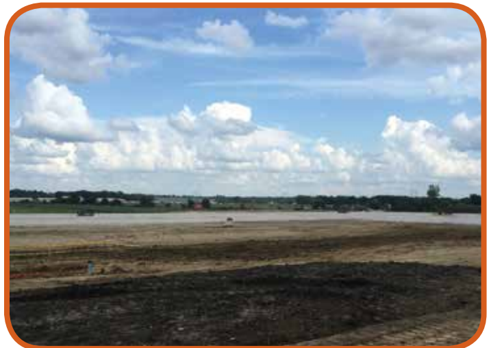
Future home for Baker Group's new complex in Ankeny
