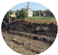
..... Corell widening the road at 156th Street in Urbandale. .....
