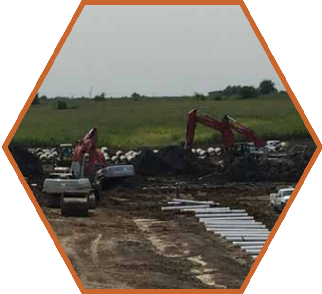
The Underground Company placing pipe at a new development in Urbandale.
