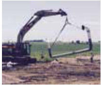
..... Brother Maurice Kerns working for Michels Pipeline in Marshall County. .....
