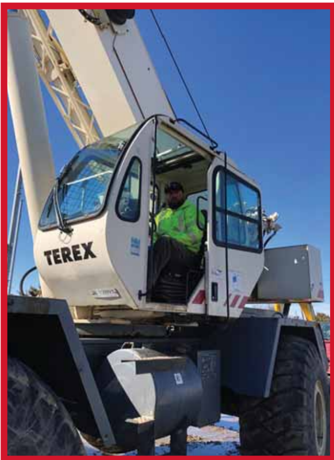
Brother Braxton Thompson operates a rt crane for ACE Construction at the Clive public safety facility
