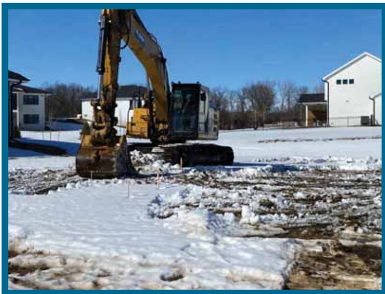
Brother Shane Herr prepping for a basement dig for Elder
