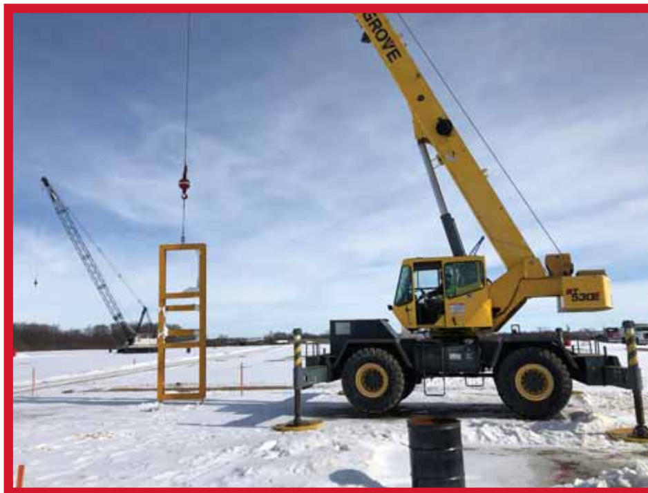
Apprentice Tyler Sylvester operating a crane at the Local 234 Training site
