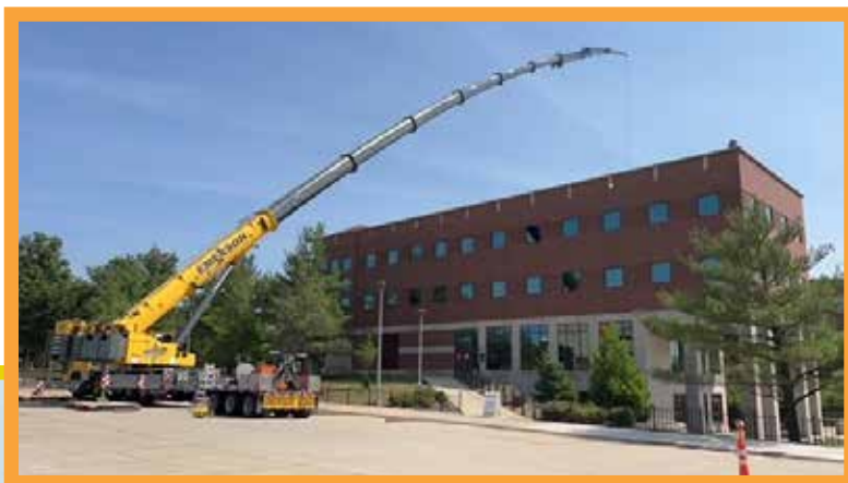
Brother Chad Emerson operates a Grove 275 ton crane and Brothers Kyle Ohrt, Grant Ries and Jake Salisbury are riggers for Emerson Crane setting an air unit for UNI in Cedar Falls
