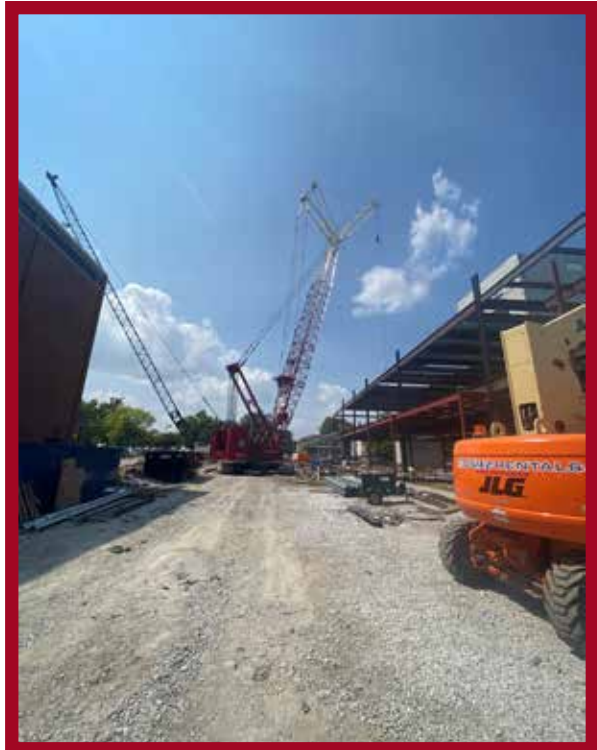
Brother Bret Alexander operates a 999 Main Boom 136' & 90' luffer setting steel for Northwest Steel at Iowa State University in Ames
