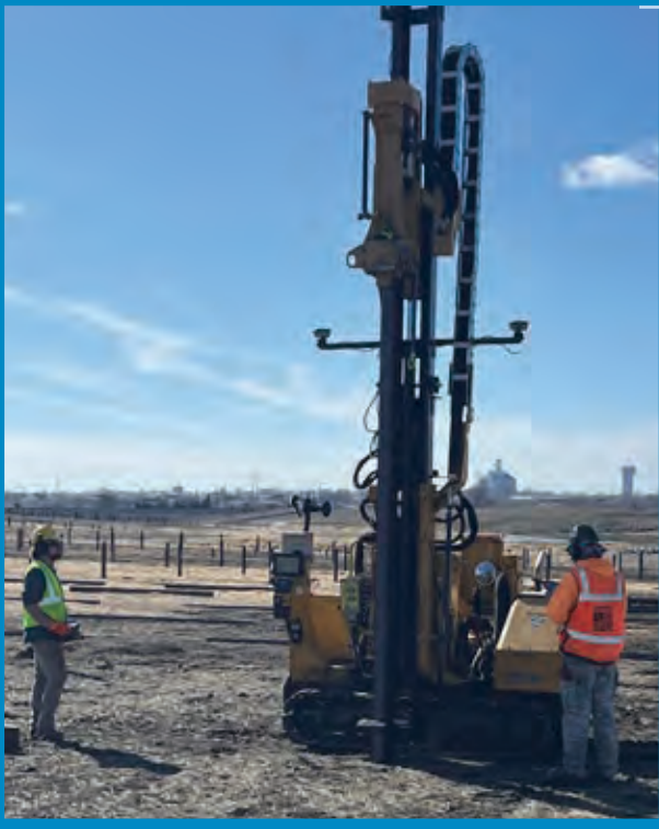
Apprentice Brodie Saville operates a PD10 Pile Driver for Azco at the Solar Farm in Creston
