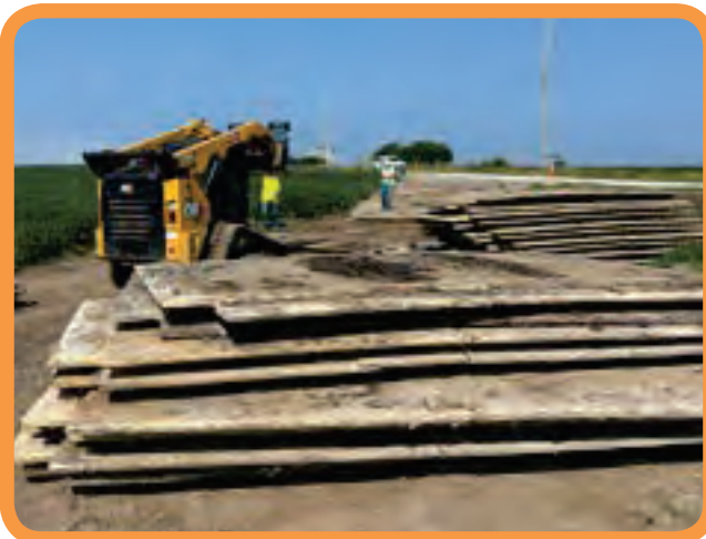
Sister Callie Faulkner and Apprentice Debra Hirth spot for Apprentice Joey Snyder as he operates a CAT skidloader setting truck mats for Mountain Crane outside of Collins
