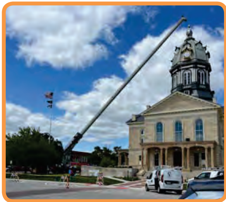
Brother Matt Mann operating a 275 ton AT installing new clocks in the Madison County Courthouse in Winterset (Not shown in the pic was Brother James Reese assisting)
